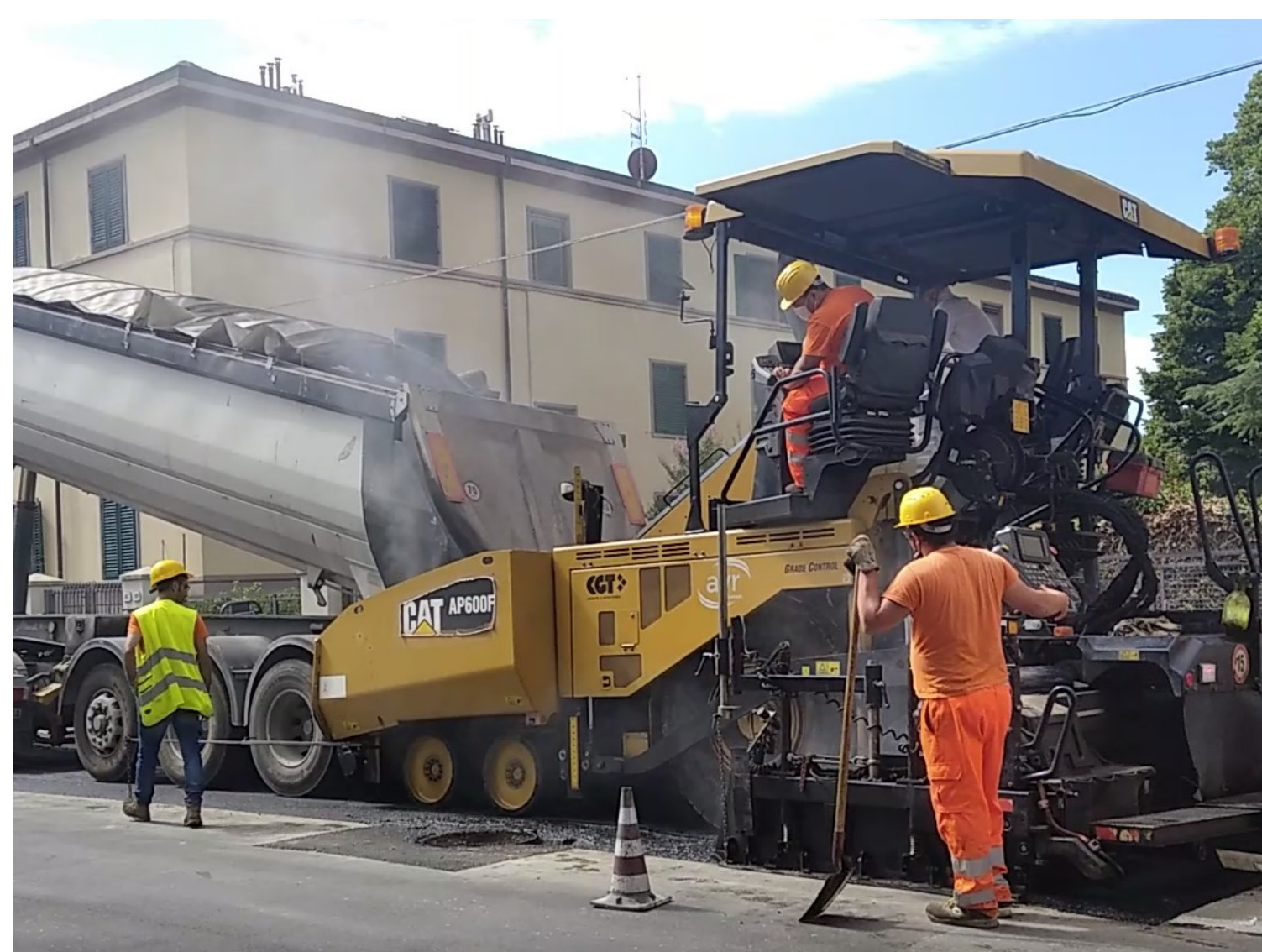
Laying a new asphalt
