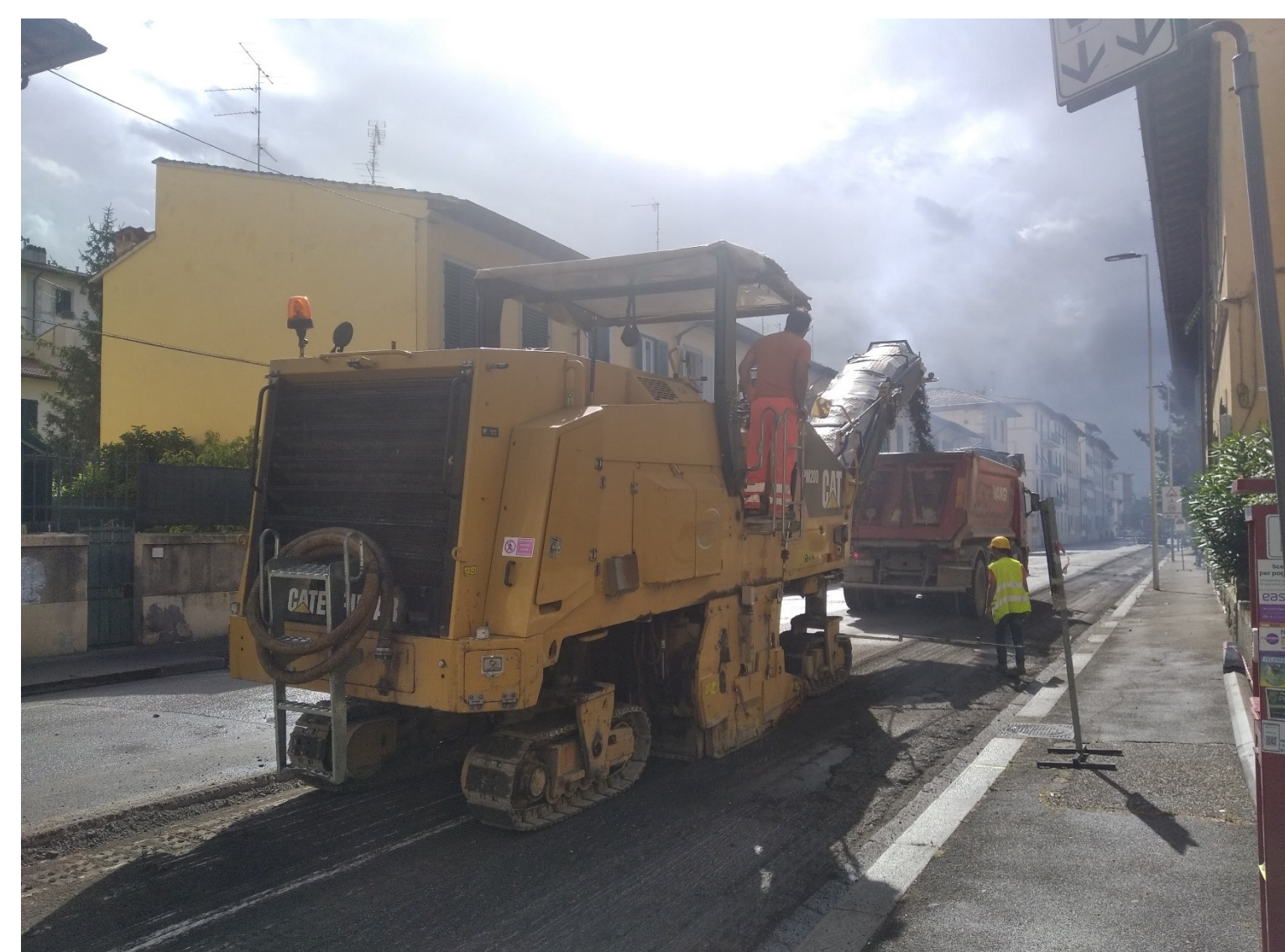
Asphalt removal
