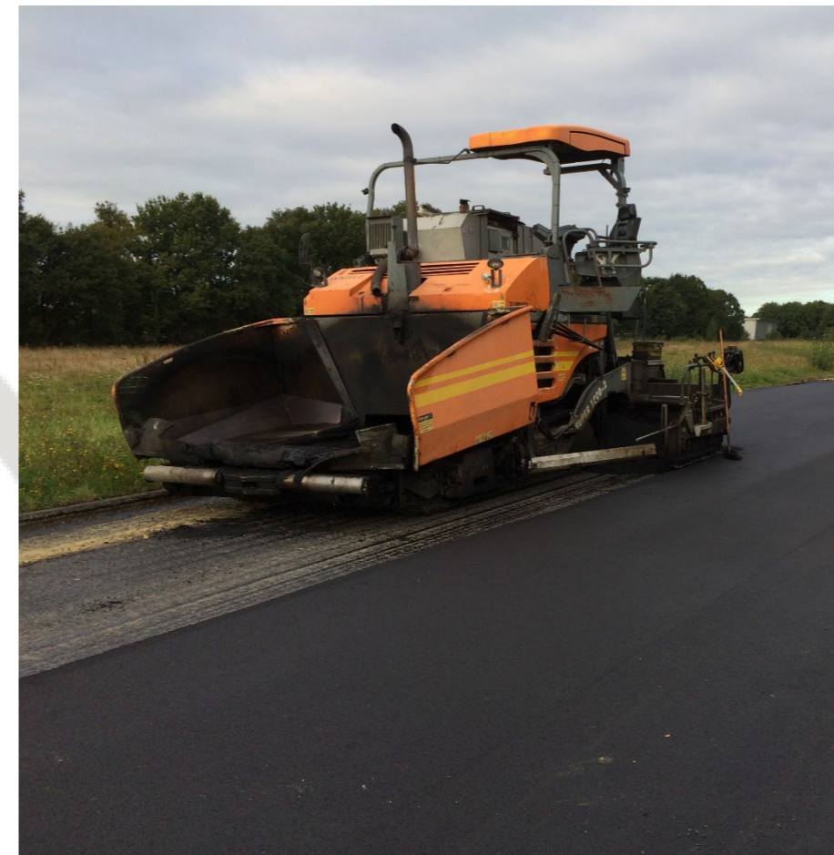
Asphalt implementation: underlayer (left), top layer in BBTM 0/6 (right)
