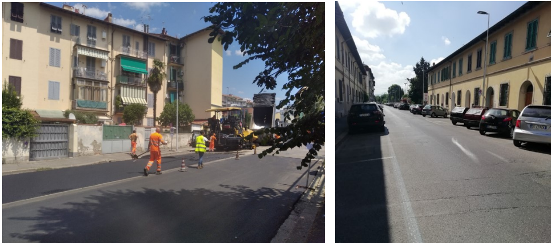
Figure 2 - The re-pavement of the pilot street
